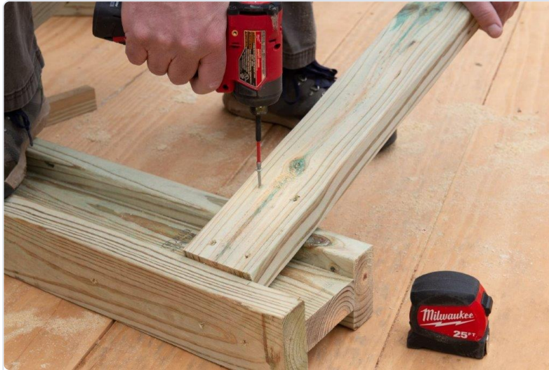
Fig. 5. Driving screws through the leg into the I-beam. Photo: The Home Depot.
