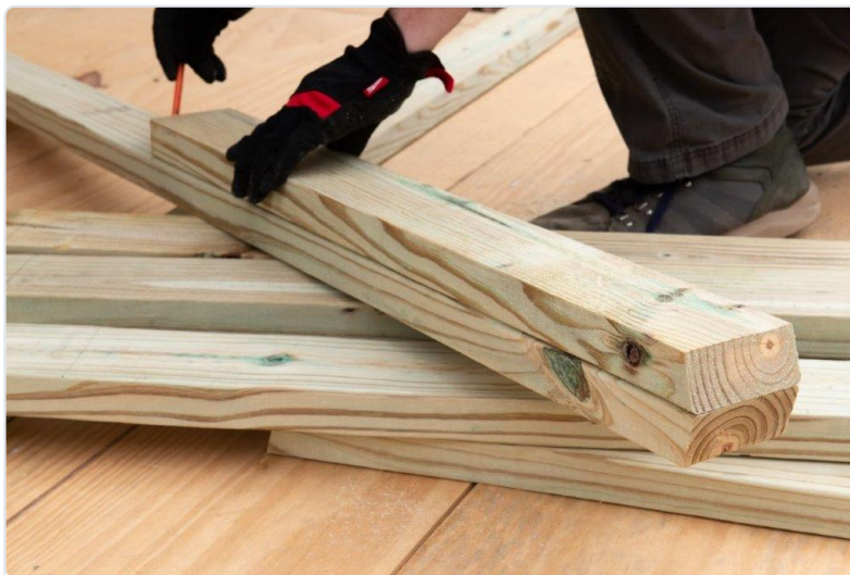
Fig. 2. Measuring a board before cutting it into a sawhorse leg. Photo: The Home Depot.
