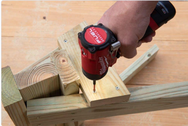
Fig. 7. Screwing gussets to each side of the sawhorse. Photo: The Home Depot.
